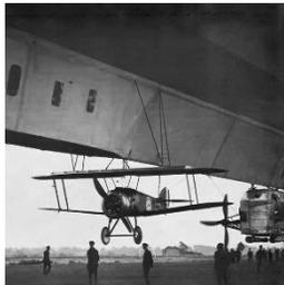
**A Sopwith 2F.1 Camel secured under the British HM Airship 23r**
